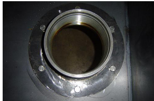
Figure 1 Well Head Flange
